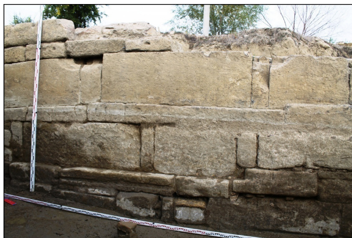
Fig. 10. The Rubas fortification. Monumental defensive wall; western facade; central section. View from west. 2017
