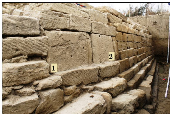
Fig. 12. The Rubas fortification. Monumental defensive wall; eastern facade. 1-2 – stone blocks with carved images. View from south-east. 2017
