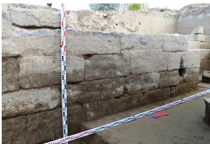
Fig. 11. The Rubas fortification. Monumental defensive wall; western facade; southern section. View from north-west. 2017
